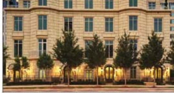
Regency Row features custom-designed doors, canopies and hand-forged carriage lamps from Putter Iron Works.
