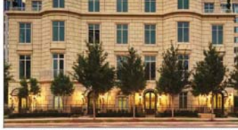
Regency Row features custom-designed doors, canopies and hand-forged carriage lamps from Putter Iron Works.
